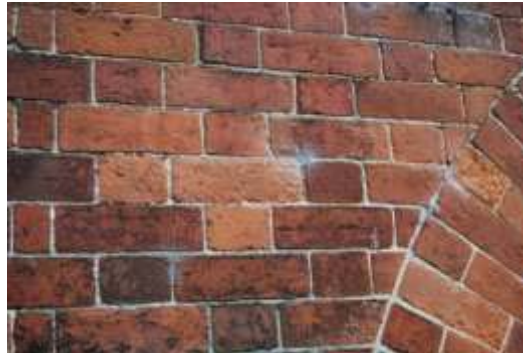
Red brick wall, former stables, Areley House
