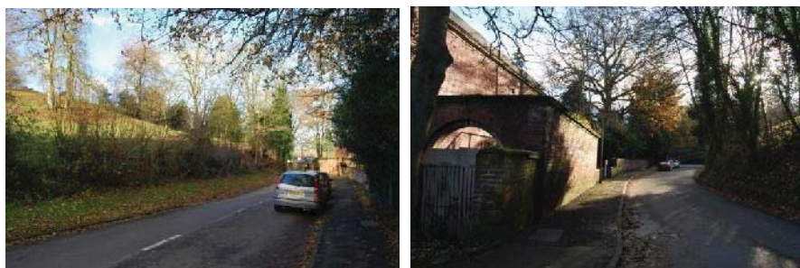
Views of Areley Lane close to Dunley Road junction
