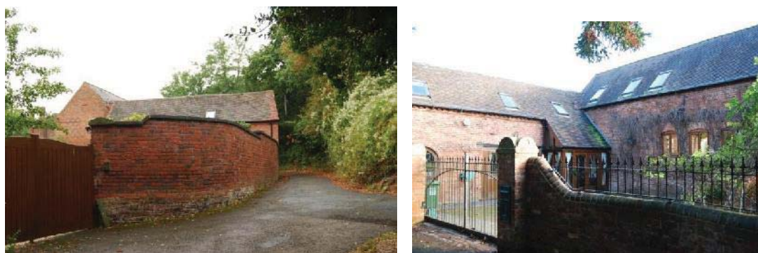
Former agricultural barns, now dwelling, Lower House Barn
