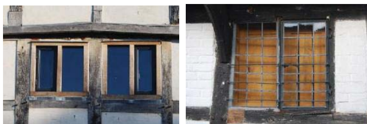
Modern timber casements and historic metal casements at Church House
