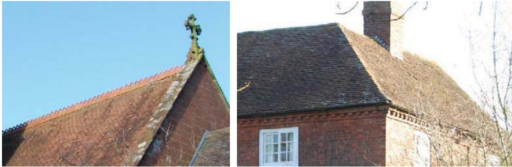
Clay roof tiles on the church and The Lower House
