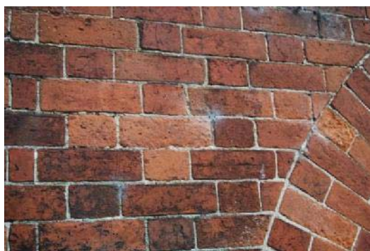
Red brick wall, former stables, Areley House
