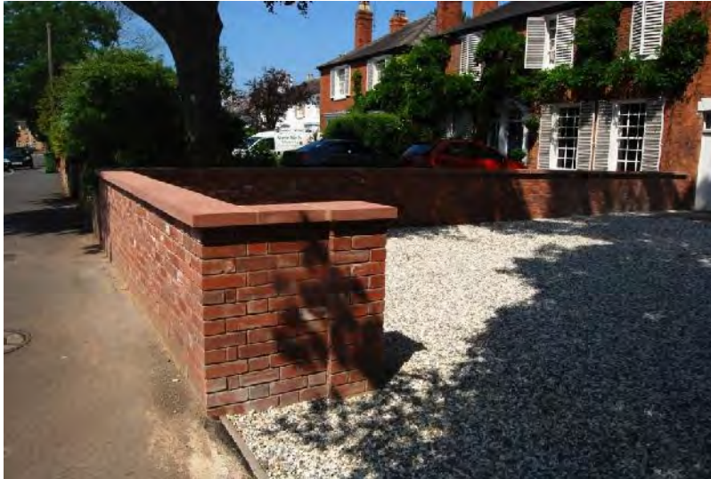
New wall built using traditional materials
