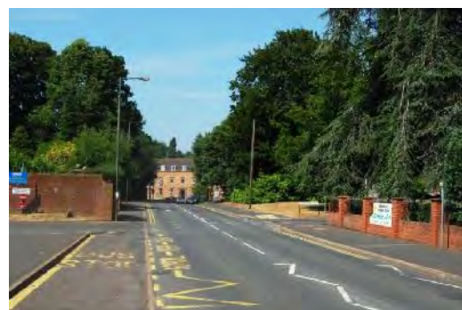
View towards the Police Station
