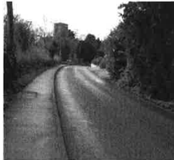
Standard tarmacadam used for both roads and pavements
