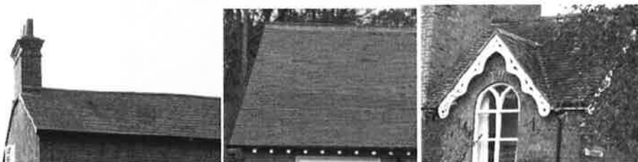
Examples of the roofing materials and colours found within the Area
